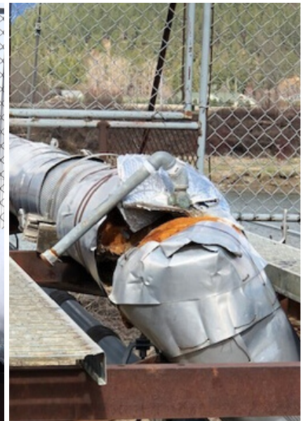
Insulation to be Replaced
