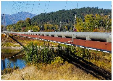
The Straights (6 ft. sections) were installed after the pipe was pulled through the Pipe Saddles
